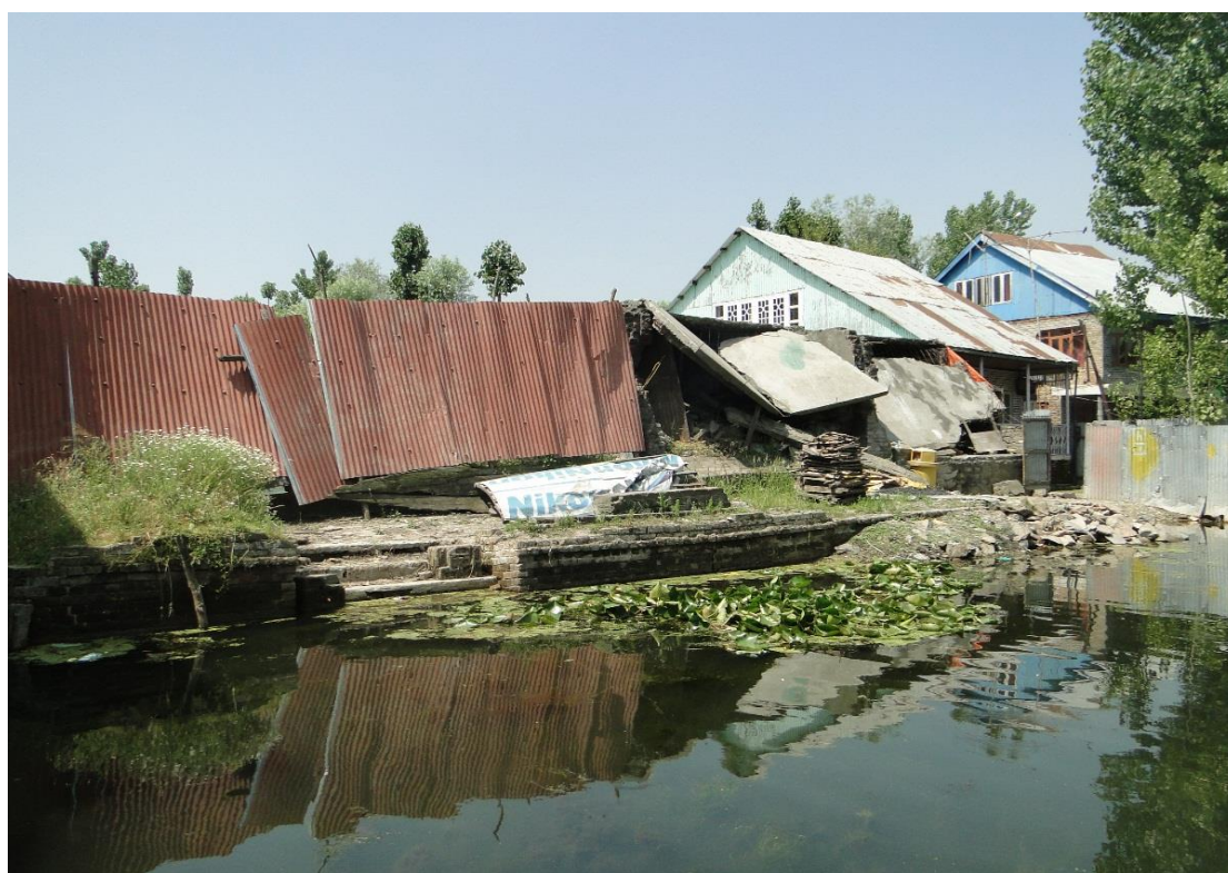
Fig.43: Demolition works in Gagribal Basin of Dal Lake
