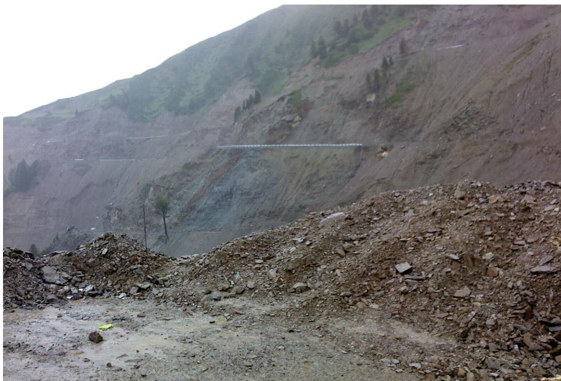
Fig.46: Highly Landslide prone area in Mughal Road
