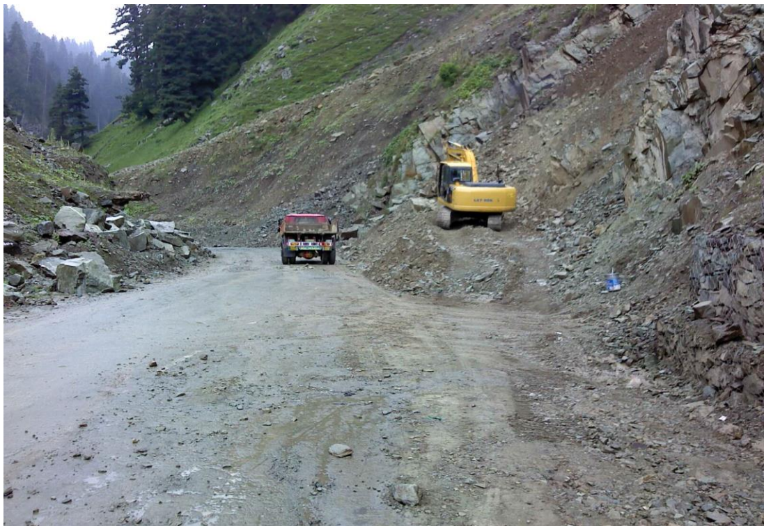
Fig.45: Landslide clearing work in Mughal Road
