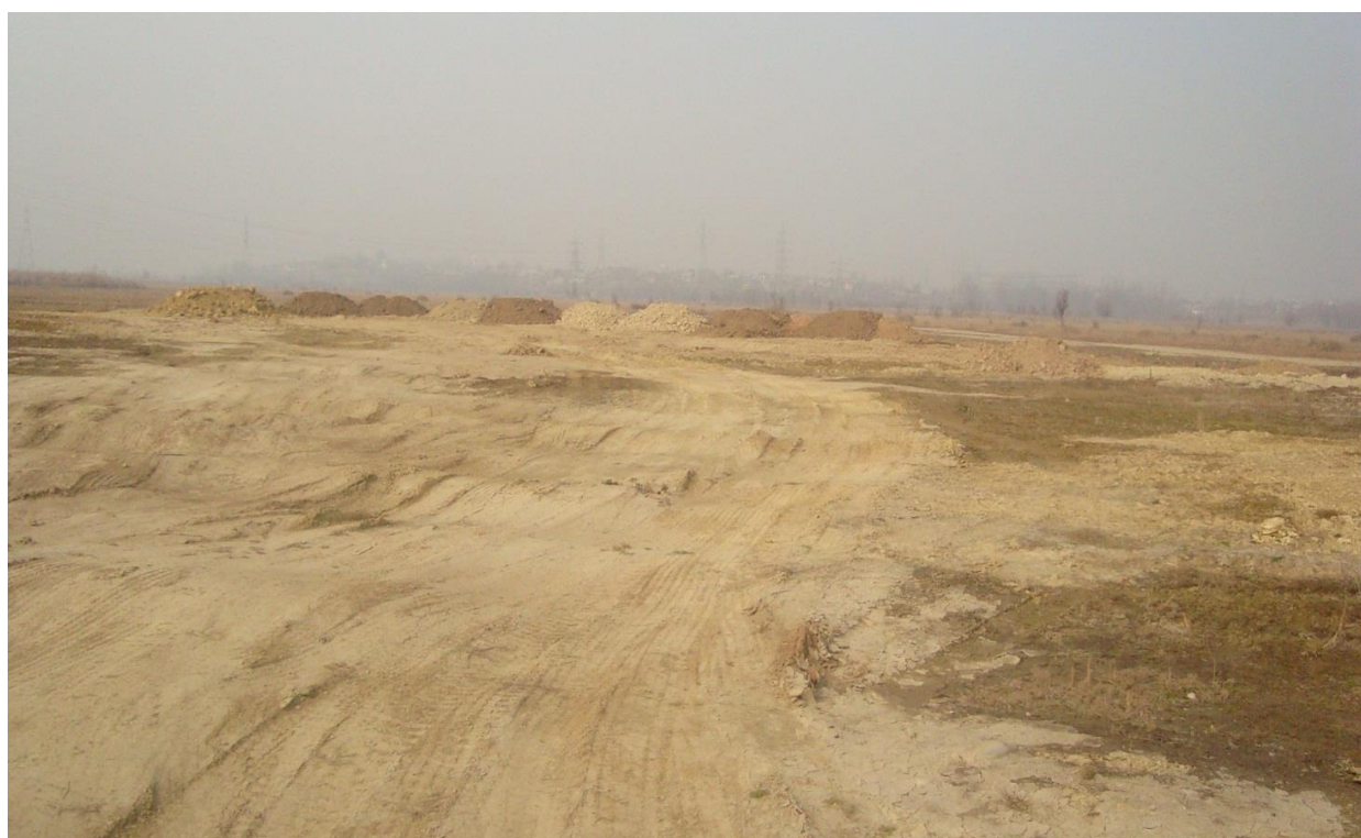
Fig.52: Landfilling works going on in Rakh-i-Arath
