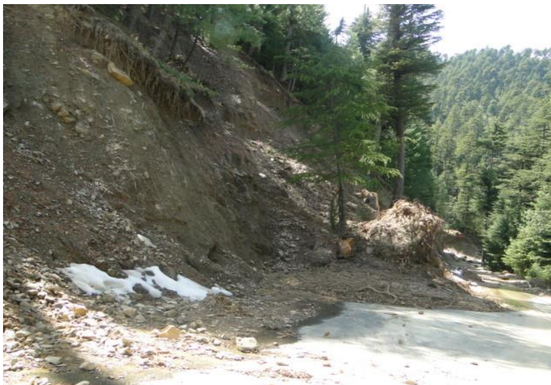
Fig.40: Batote-Kishtiwar Road blocked due to landslide
