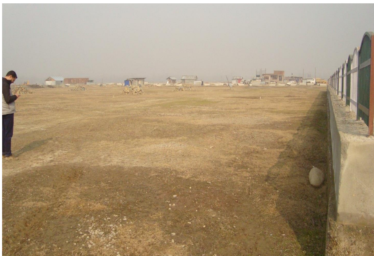
Fig.51: Construction works in Rakh-i-Arath
