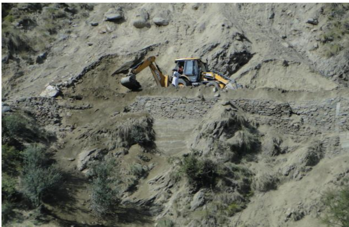
Fig.42: Landslide clearing work on Batote-Kishtiwar road
